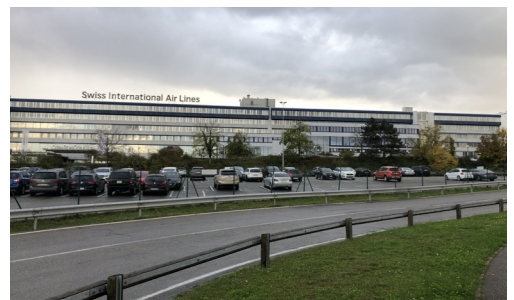
Technical Due Diligence Business Building EuroAirport Basel Mulhouse
